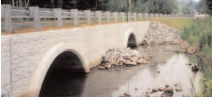
Precast concrete short-span bridges have many advantages over competing materials:
