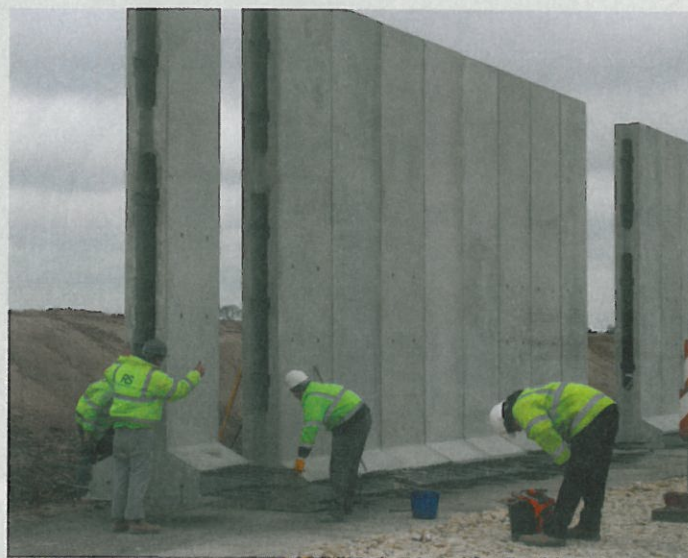
Shuttabloc combines precast concrete walling with in-situ pouring
